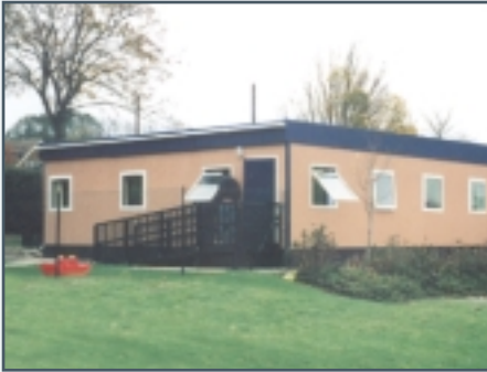
Standard Modular building
